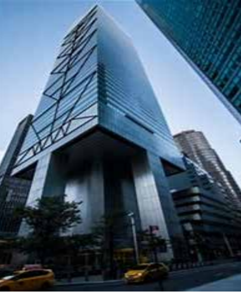
59 floors Could Have Topped Built in 1977 for Citibank, it is 915 feet (279 m) tall and has 59 floors with a combined 1.3 million square feet (120,000 m2) of office space. The building was designed by architect Hugh Stubbins, associate architect Emery Roth & Sons, and structural engineer William LeMessurier. A tuned mass damper (TMD) is a device consisting of a mass, a spring, and a damper that is attached to a structure in order to reduce the dynamic response of the structure.
